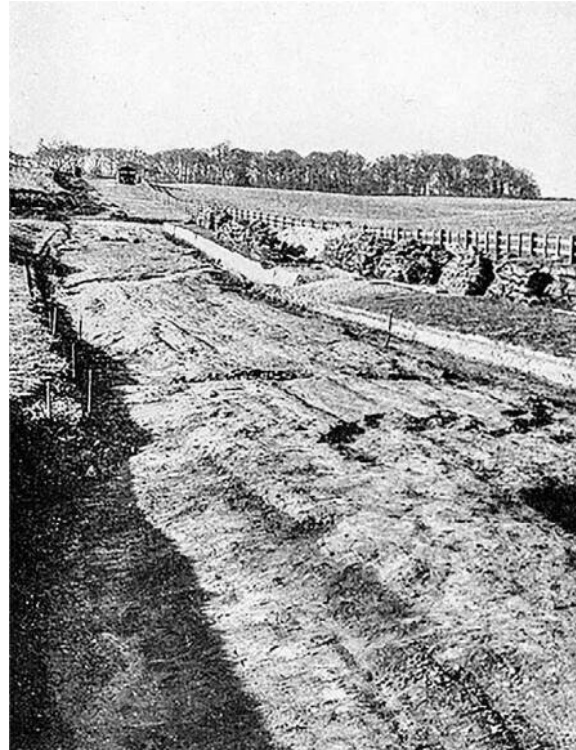
FIG. 1. London-Lewes Way, a Roman road near Holtye, Sussex, paved in iron slag (Margary 1965, frontispiece).
