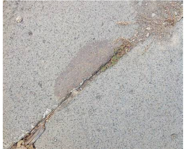
FIG. 9. Example of Type 3, staining at pour point, Supplementary Table, ID_432, Via Stabiana.
