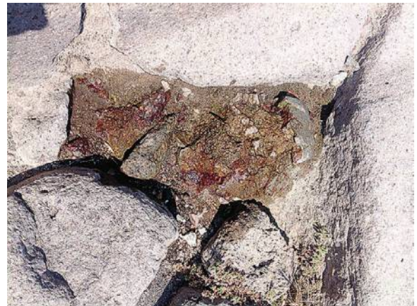
FIG. 16. Example of Type 6, repair with composite materials, Supplementary Table, ID_422, Via Stabiana. Note that the deposit (ca. 40 cm x 20 cm) includes large stones and that it fills a large gap between paving stones.
