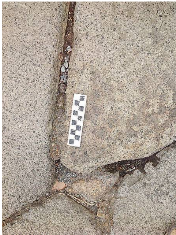
FIG. 7. Example of Type 2, solid with staining, Supplementary Table, ID_157, Via della Fortuna. Note the ferric materials filling the junction between paving stones and the stains in the pockmarks on top of one paving stone.
