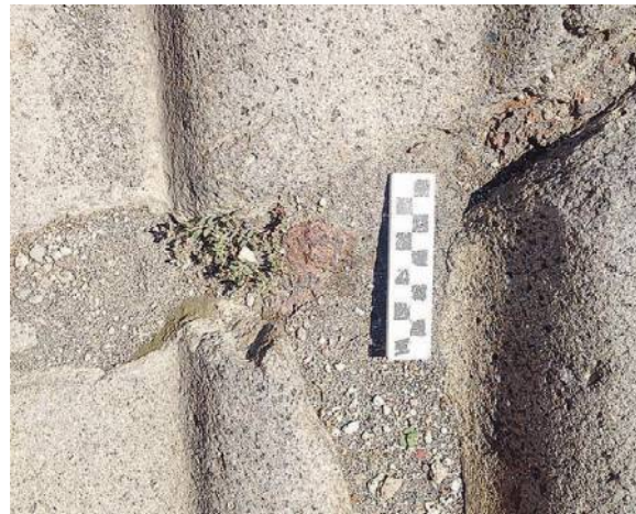
FIG. 4. Example of Type 1, solid without staining, Supplementary Table, ID_297, Via Stabiana. Note the solid iron at the bottom of a deep rut and degraded iron filling between paving stones.
