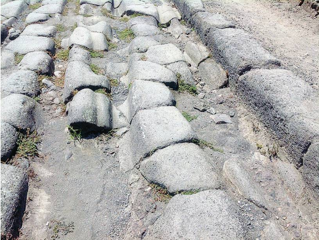
FIG. 14. Deeply rutted section of Via della Fortuna containing remnants of many repairs.
