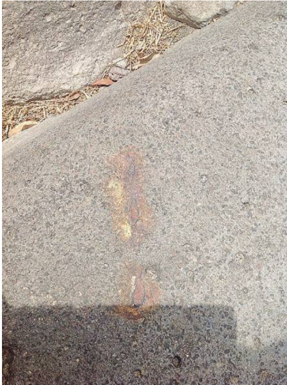
FIG. 8. Modern example of Type 2, solid with staining, Supplementary Table, ID_004, Via Stabiana. The stains were made by the feet of modern steps that have now been removed.
