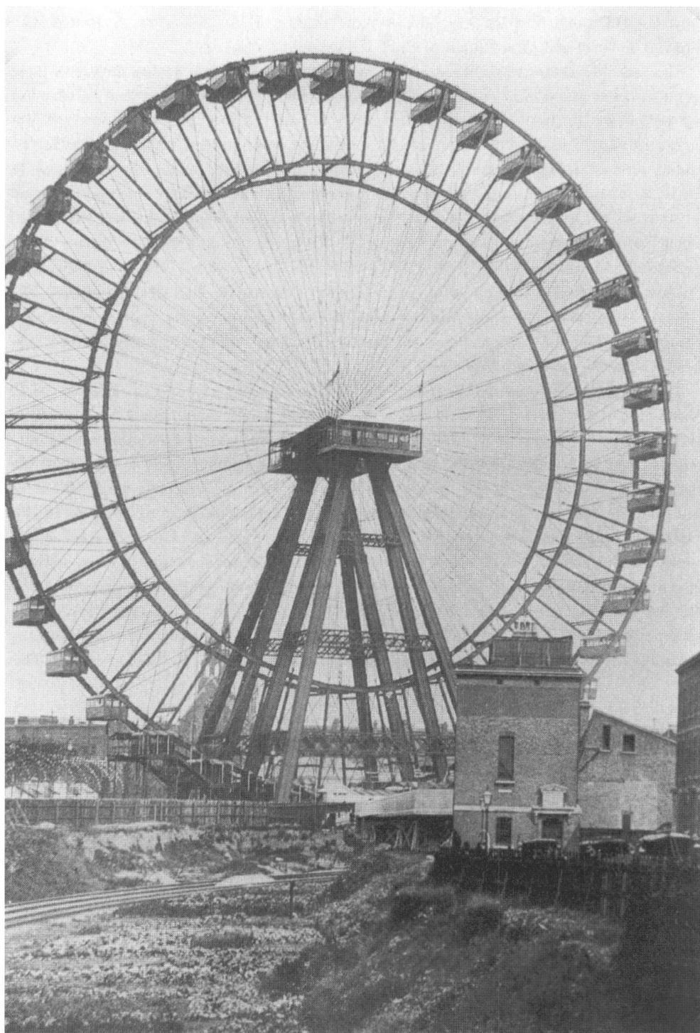
Fig.95 The Great Wheel at Earl's Court which was built in 1895 by Maudslay's and powered by one of their marine engines. ( L. Ince )
