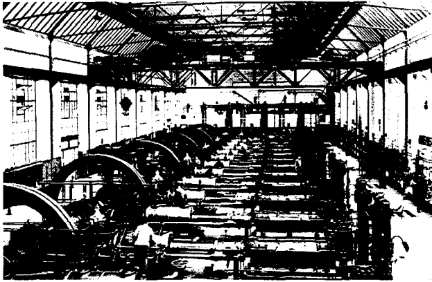
Fig. 55. High pressure lye pumps for gas purification.
