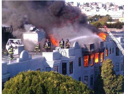
(a) Five-Alarm Fire at 1502 Golden Gate Ave, 2011
