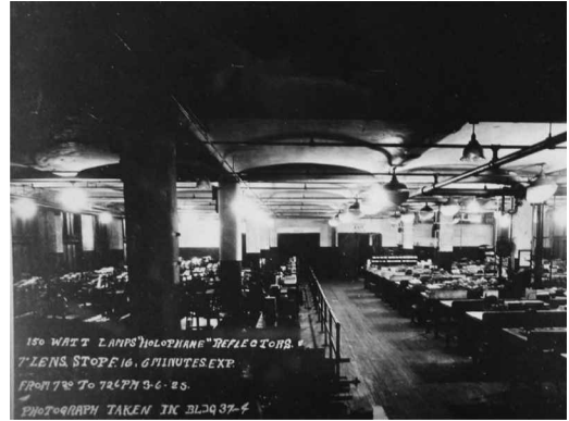
Figure 10. Jack Shell and Spring Inspection Room at Night with 150 Watt Holophane Reflectors. Photograph taken in 1925. Photograph by Marty Labnos. Credit: Charles D. Wrege Collection, History of Management Photographs, Kheel Center, Cornell University.
