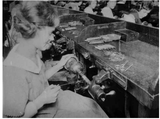
Figure 6. Coil Winding Task. Photograph taken in 1925. Photographer unknown. Credit: Charles D. Wrege Collection, History of Management Photographs, Kheel Center, Cornell University.
