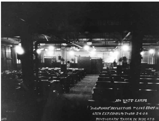
Figure 9. Coil Winding Room at Night with 150 Watt Holophane Reflectors. Photograph taken in 1925. Photograph by Marty Labnos. Credit: Charles D. Wrege Collection, History of Management Photographs, Kheel Center, Cornell University.
