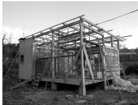
Figure 7 Test Cells in construction.
