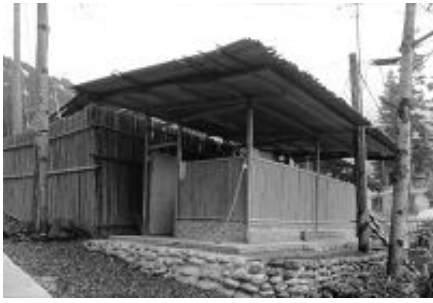
Figure 5 Photograph of a rebuilt public kitchen of the Thao tribe in Brawbaw village, Nan-tao County, Taiwan, which was reconstructed by bamboo-weaving roof, rib-frame structure, bamboo-weaving wall and rock-brick foundation.
