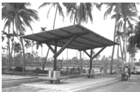
Figure 2 Photograph of a new pavilion in Zhen-ban village, Ping-tong County, Taiwan, referred to the art of composition from structural frame made of bamboo, which was used by aboriginal Shao tribes.
