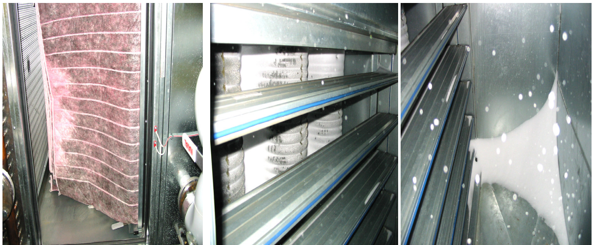
Figure 2 The fine filter chamber is located in the left, the needle heat exchanger is in the middle and the cold air chamber is located in the right side.
