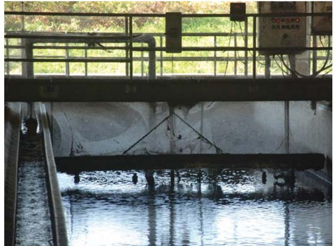
Fig. 8. Webbing beneath traveling bridge.
